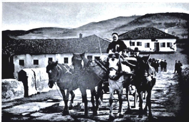
ON A FRONTIER BRIDGE.
